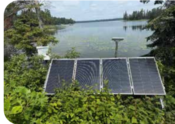
Four solar panels supplied power for the autonomous Loon Cam system.
